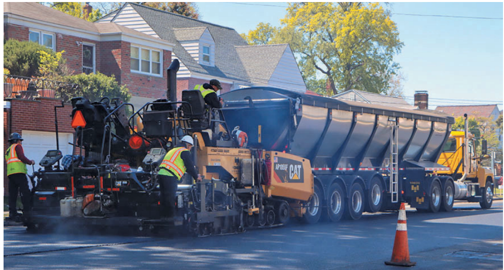
Yonkers Contracting paving using hot mix asphalt with Anova® Rejuvenator produced at Peckham's Bronx plant - Madison Kappel - Peckham Industries.
