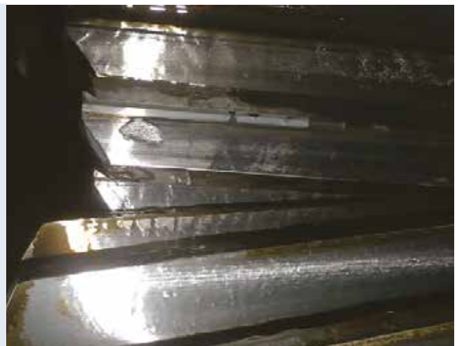
Figure 8 Visible corrosion at the tooth flank
